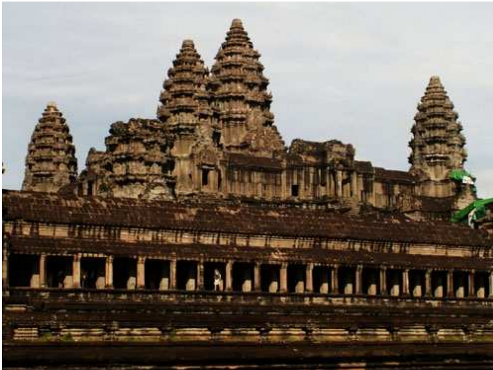
Example of World Heritage building with well-integrated INDELEC Lightning protection System installed (Angkor Vat – Cambodia)
