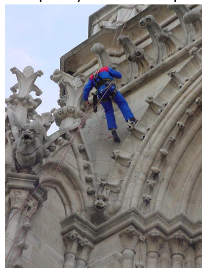
Down-conductor fixing on Notre Dame de Paris and its famous gargoyles
