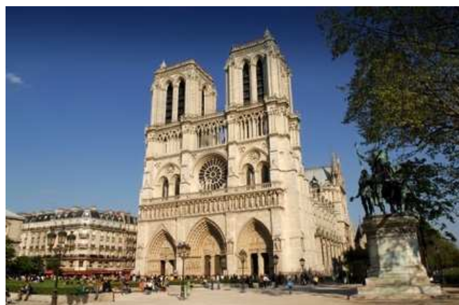
Installation of the Prevelectron ESE air terminal on Notre Dame de Paris cathedral: The air terminal is not visible for visiting tourists from ground level (western facade).
