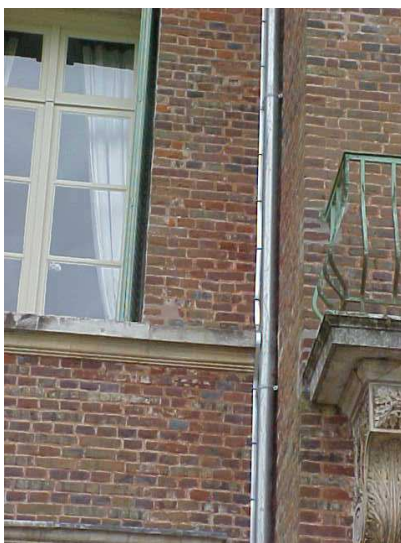
Example of conductor routing along a gutter
