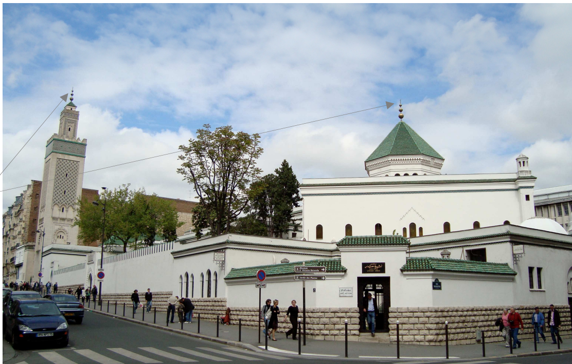
Grande Mosquée de Paris (largest mosque in France and the third largest in Europe) protected with two Prevectron MH air terminals (Paris – France)
