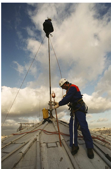
Daijingu Shrine (Japan) protected by a "hidden" INDELEC lightning air terminal
